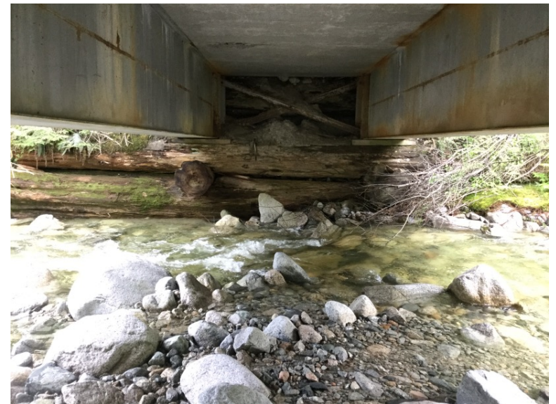
Right Bank Abutment when facing downstream
