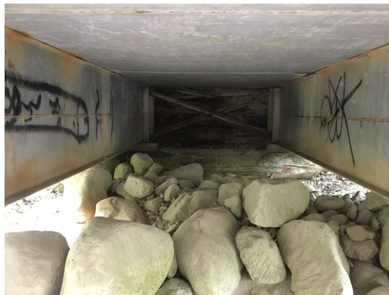
Left Bank Abutment when facing downstream
