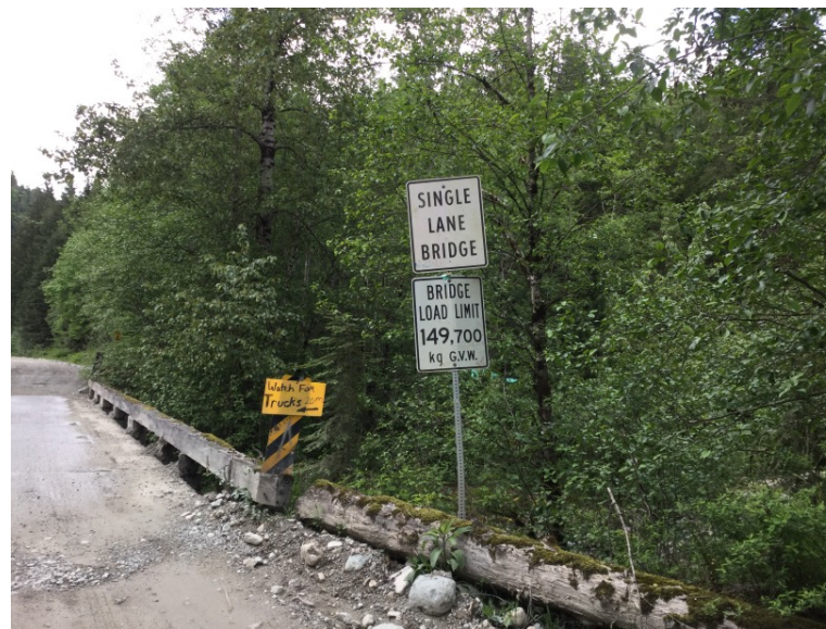
Load Rating Sign
